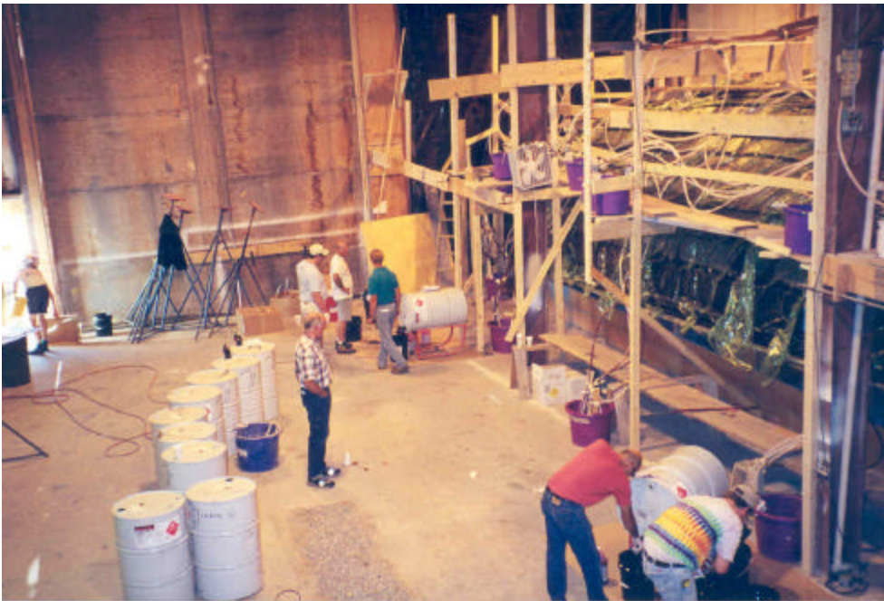
Vinylester resin was applied by SCRIMP infusion.
